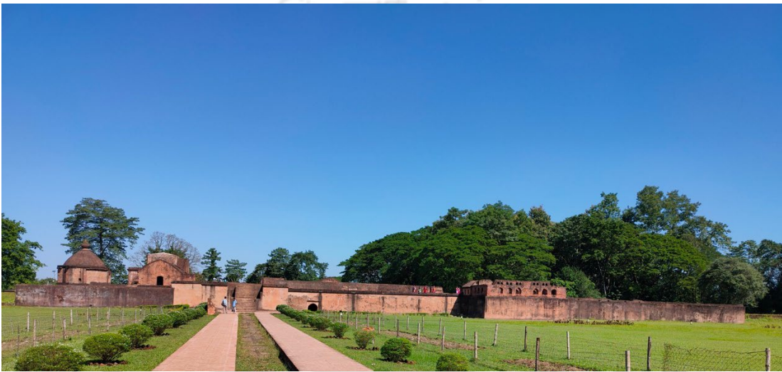
Appx A Fig. 1. 4 Talatal Ghar, Sivsagar- Photographs of various sections of the monuments
