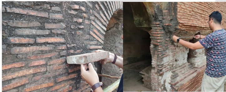
Appx B Fig. 1. 2 Observation of early brick with the custom brick sizes
