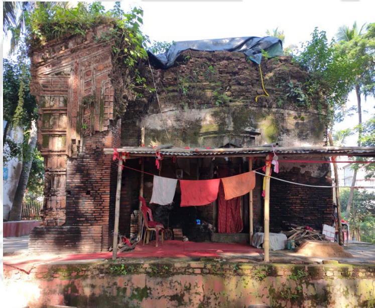
Fig 2. 15 Front section of Namath Kali, Nilachal Hills, Guwahati.
