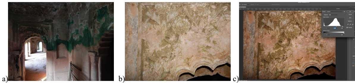
Fig. 3. 2 a) Normal lighting inside the Talatal Ghar, Sivasagar; b) Lightning setup for visibility; c)Photo enhancement for details using editing software.
