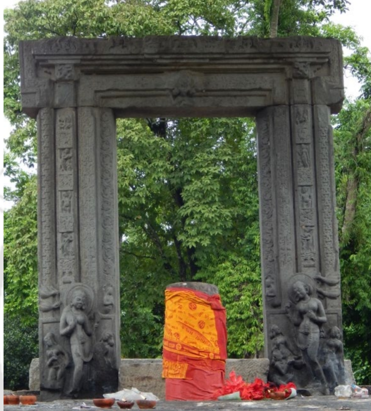
Fig 2. 8 The Dah-parvatiya temple stone door, Tezpur, Assam.
