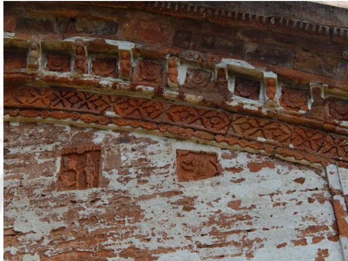
Fig. 4.1 Variations of terracotta plaques on the side wall, Ghanasyam House, Sivasagar, Assam.
