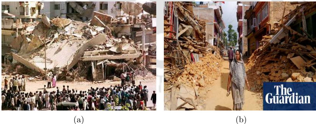
Figure 1.1: Devastating effects on buildings due to (a) Bhuj Earthquake, 2001 and (b) Nepal Earthquake, 2015. photo courtesy : Solomon and Haynes (2018); Jones (2015)
