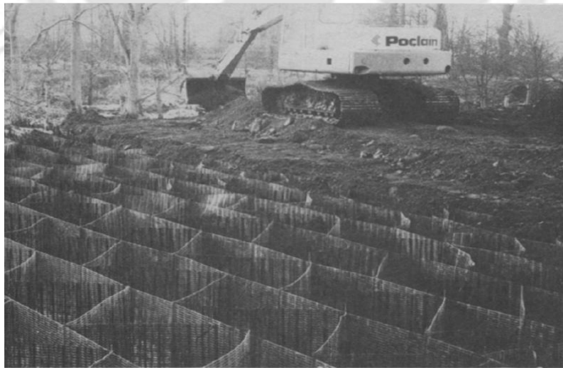
Fig. 2.1 Geocell mattress (Bush et al. 1990)
