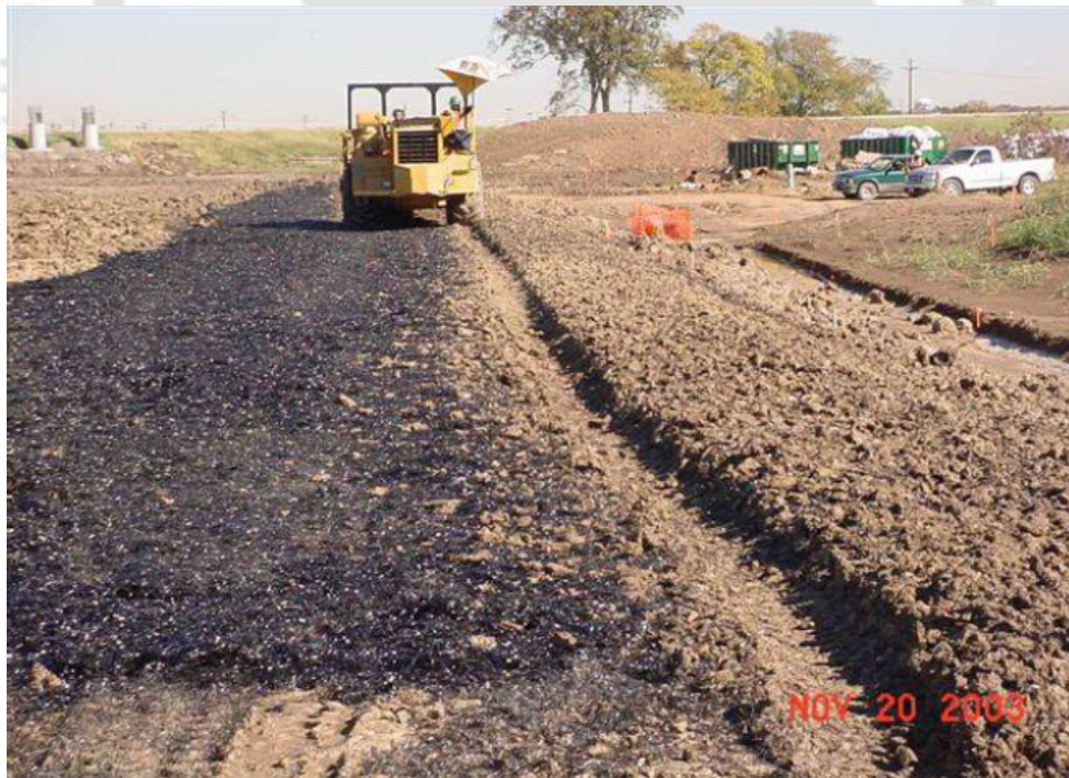
Fig. 1.9 Mixing of fiber with soil (Gregory, 2006)
