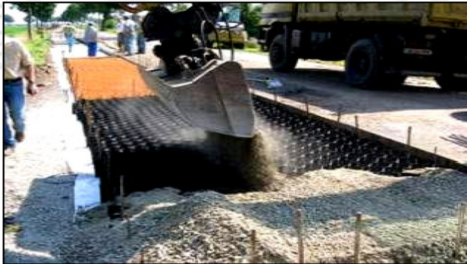
Fig. 1.5 Geocells being filled with soil (Emersleben and Meyer, 2008)
