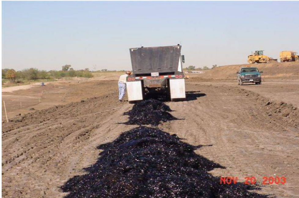
Fig. 1.8 Placement of fiber over scarified soil (Gregory, 2006)
