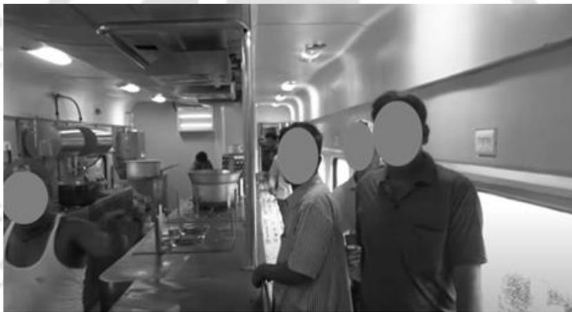
Figure 4.19. Existing condition of the air-conditioned pantry car kitchen
