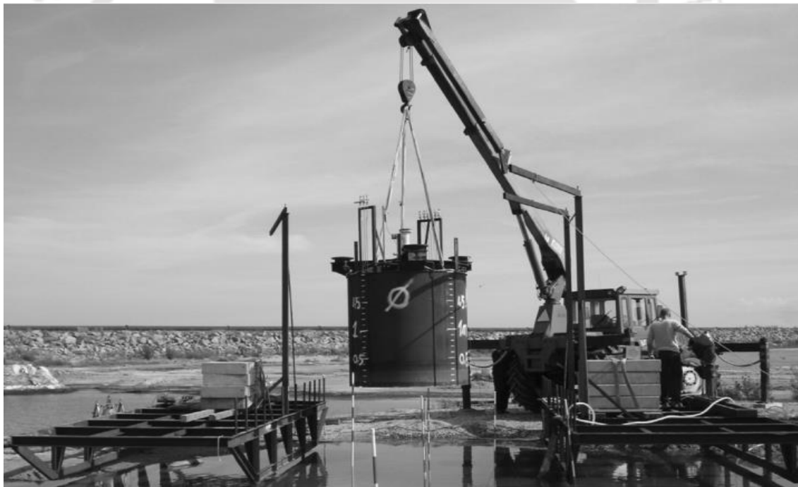
Figure C.2 Field model bucket foundation in Frederikshavn (Houlsby et al. 2005)
