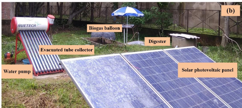
Fig. 3.6. Field-scale AD plant setup (a) schematic diagram (b) photograph.
