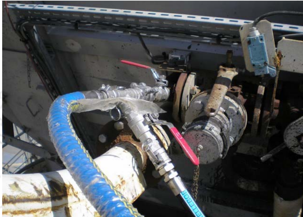
Figure 2.7: Staking of Evotherm DAT line to bitumen line (Maze et al., 2011)
