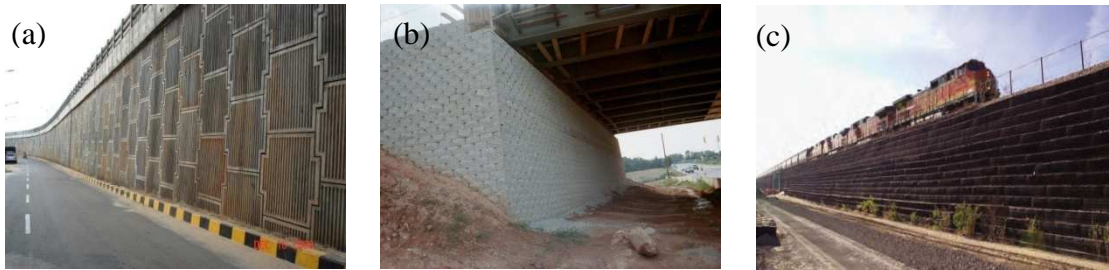
Fig. 1.1 Application of reinforced soil structures: (a) highways; (b) bridge abutments; and (c) slope stability ( www.reinforcedearth.com )
