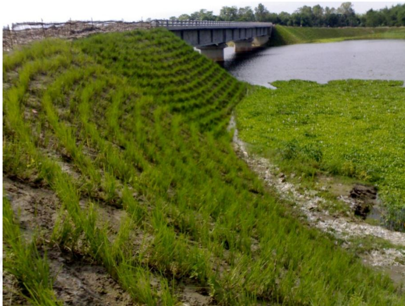
Fig. 1.1 Slope protection using vegetation for Dora bridge abutment in Assam, India ( http://www.chhajedgarden.com/blog/vetiver-planting-for-slope-stabilization/ )
