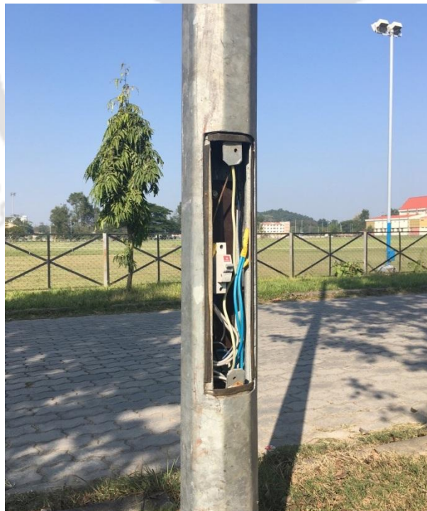
Figure 1.6: Perforation provided for electrical services
