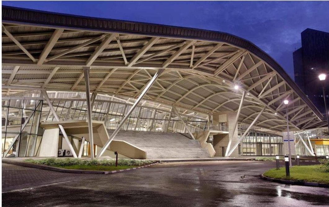
Figure 1.3: CIDCO Exhibition and Convention Centre, India (Image by www.iniiinfraengineering.com/upload_image/55.jpg )
