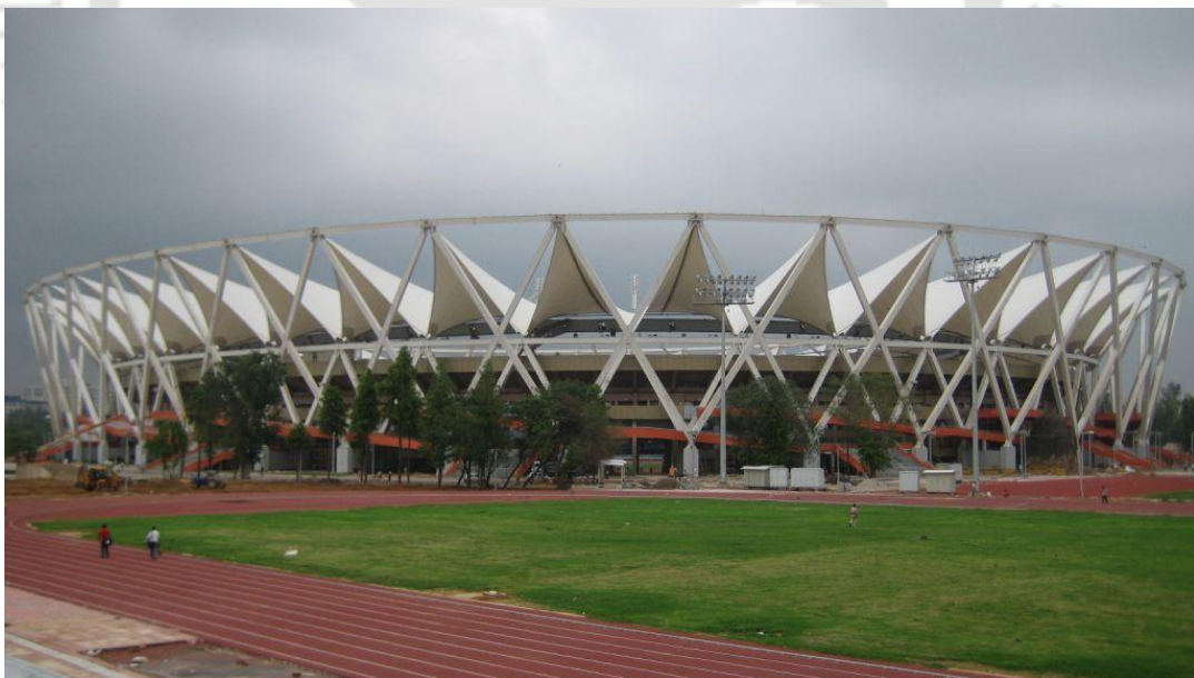
Figure 1.4: Jawaharlal Nehru Stadium, India (Courtesy: Tata Structura Tubes Division, Kolkata)
