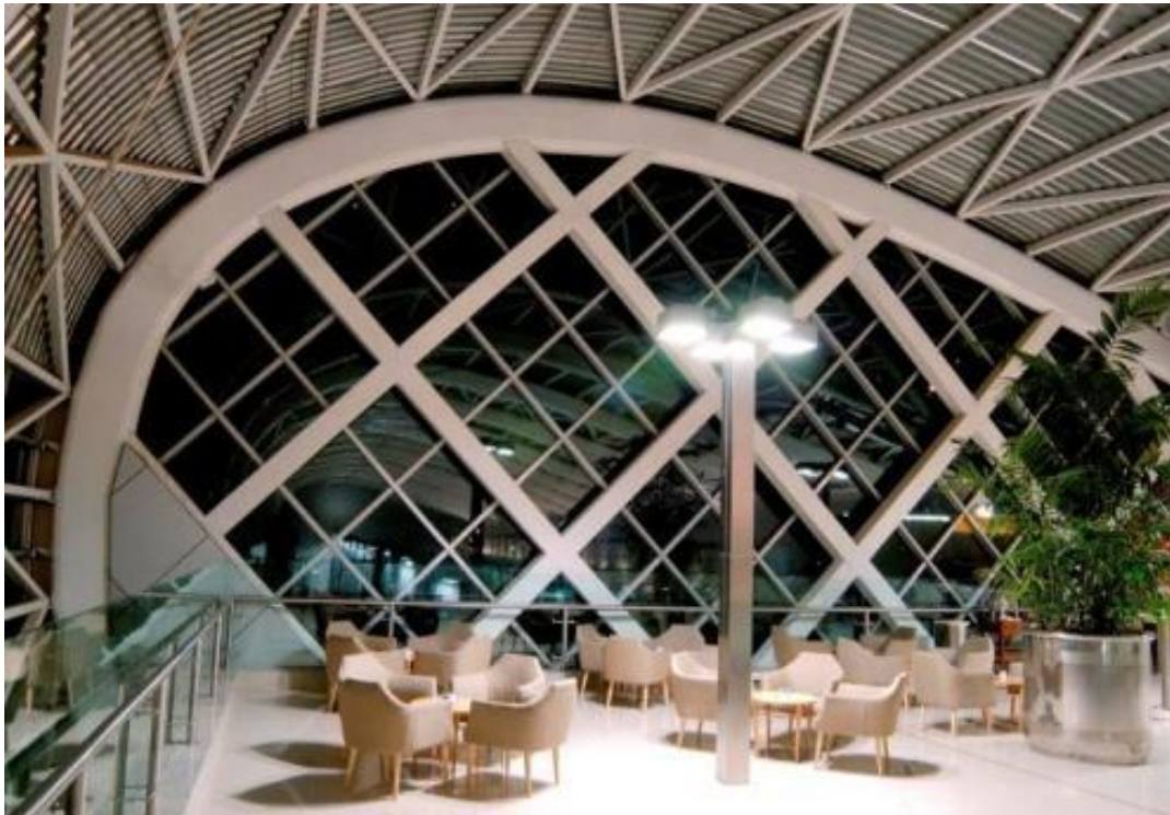
Figure 1.5: Chhatrapati Shivaji International Airport, India (Courtesy: Tata Structura Tubes Division, Kolkata)
