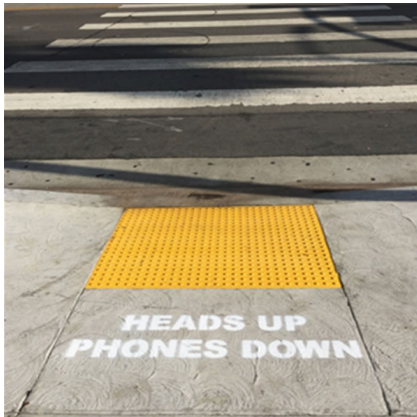
(A) Stencil reminder installed at crosswalks in California, USA (Barin et al., 2018)
