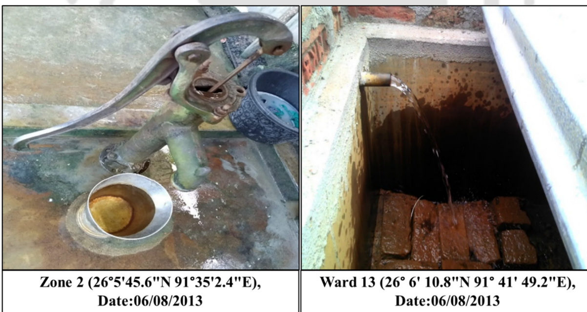
Figure 6.2: Precipitated iron besides groundwater sources.
