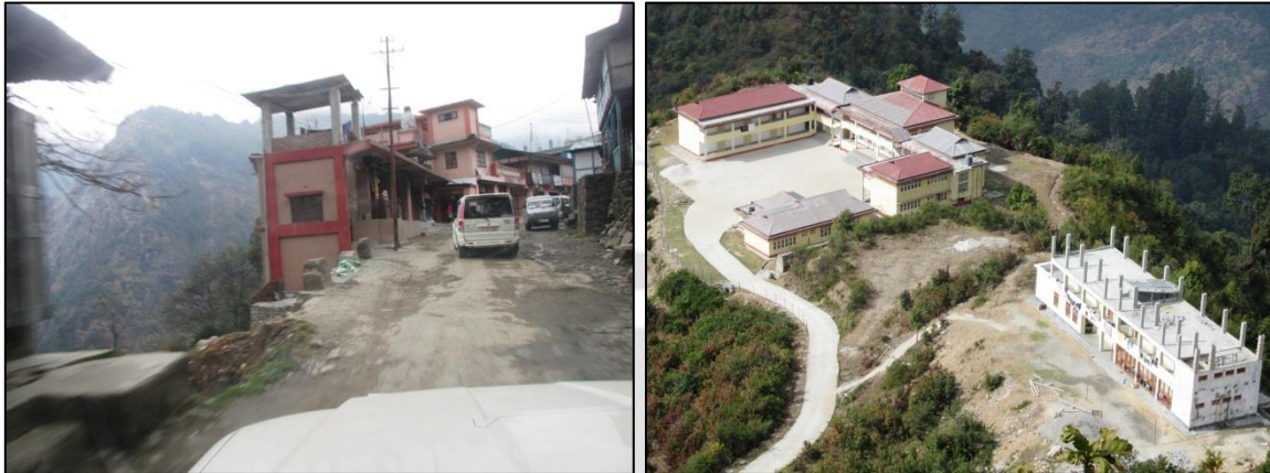
Figure 1.1 Buildings right at the verge of steep slopes (Photo courtesy: Arindam Dey, 2015)
