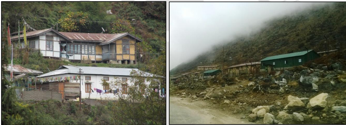
Figure 1.4 Closely spaced buildings on the hill slopes at same or different elevations (Photo courtesy: Arindam Dey, 2015)
