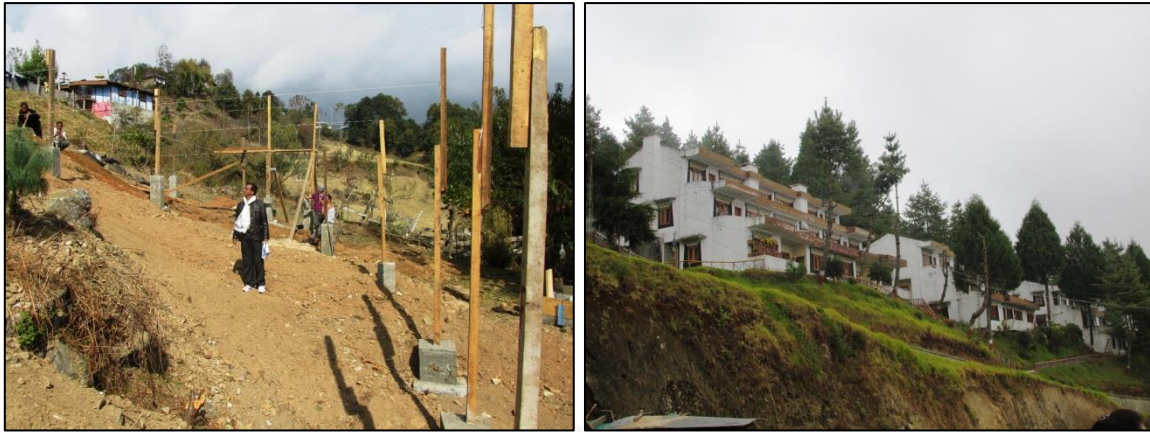
Figure 1.3 Foundation being laid and building constructed on slope face (Photo courtesy: Arindam Dey, 2015)
