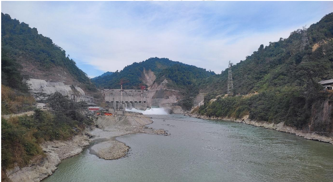
Figure 30: The under-construction dam on the river Obonori (Source: Author)
