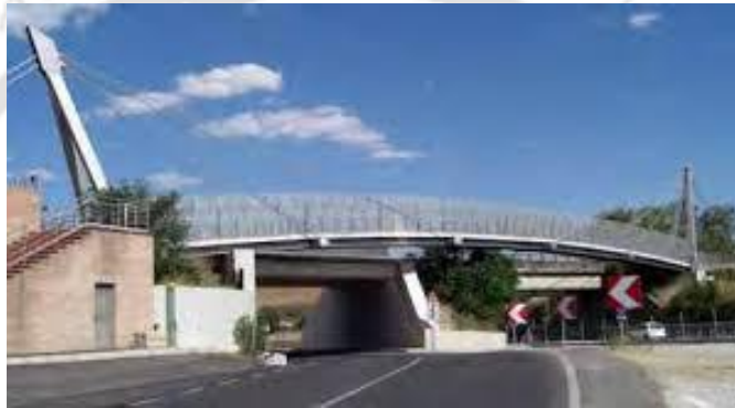
Siena Footbridge, Italy ( www.nickelinstitute.org )
