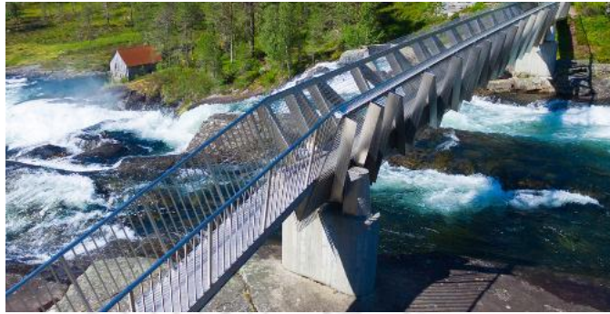
Likholefossen bridge, Norway ( www.outokumpu.com )
