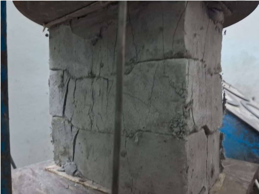
Figure 6.6: (B) Typical failure pattern (stretcher face) of FCIB prisms (triplets) under compression.
