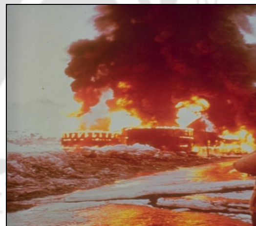
Figure 1.3: Seismic effect to industrial liquid storage tanks.
