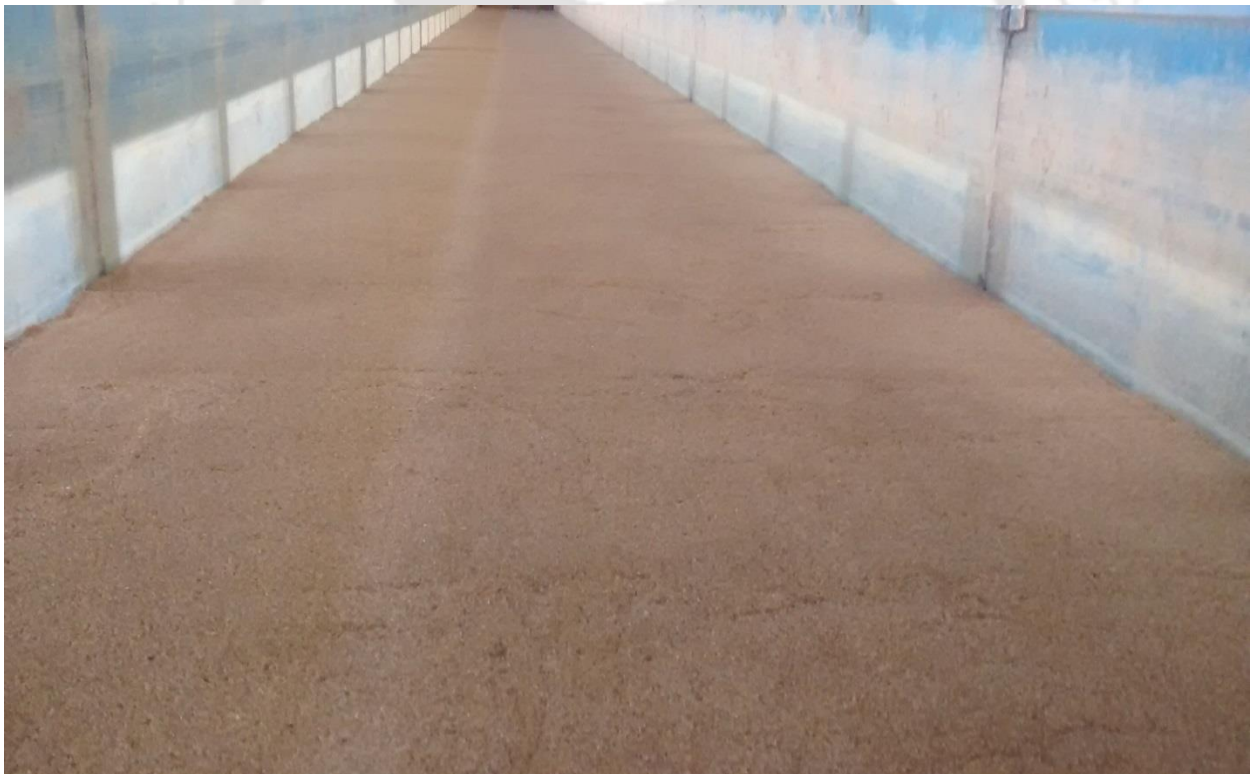
Figure 2.18: Snapshot of the channel before performing the no seepage experiments
