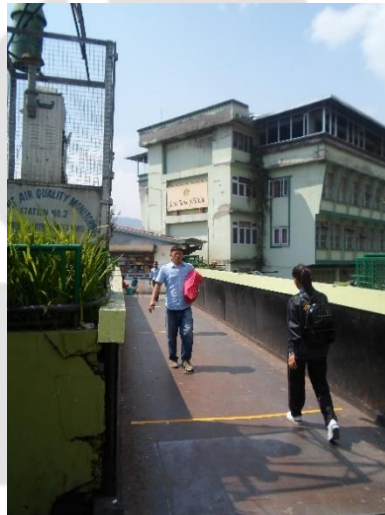
Fig. (b). STNM Hospital mid-block (F2)
