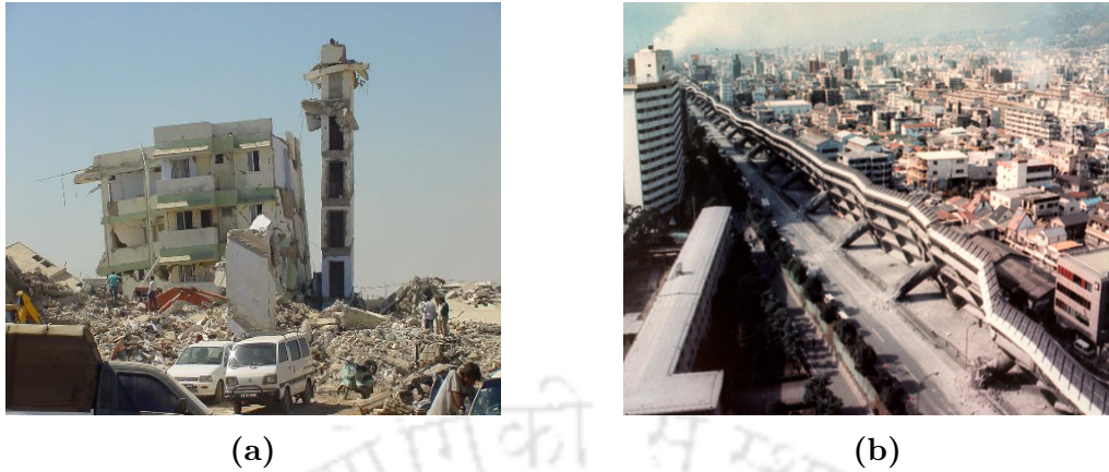
Figure 1.1: Earthquake damage of infrastructure; (a) Bhuj earthquake dated 26 th January 2001 (Source: www.nicee.org ), and (b) Kobe earthquake dated 17 th January 1995 (Source: The Wall-Street Journal)
