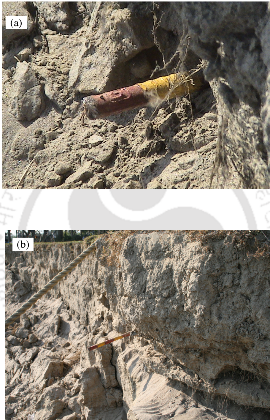
Fig. 3.18. Bank erosion measurement through erosion pins: (a) initial exposure of the pin, (b) After partial erosion of bank
