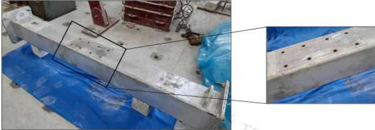
Fig. 4.8 Visual observation on panel zone and CFT column
