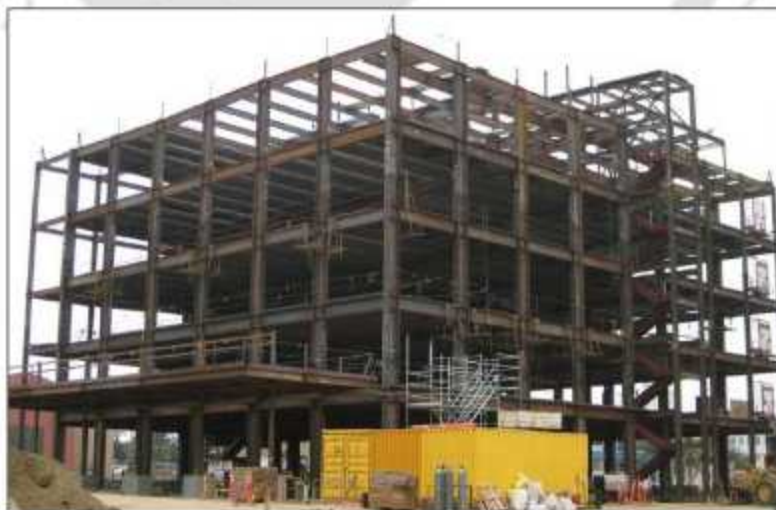
Fig. 1.1: Steel moment resisting frame [1]
