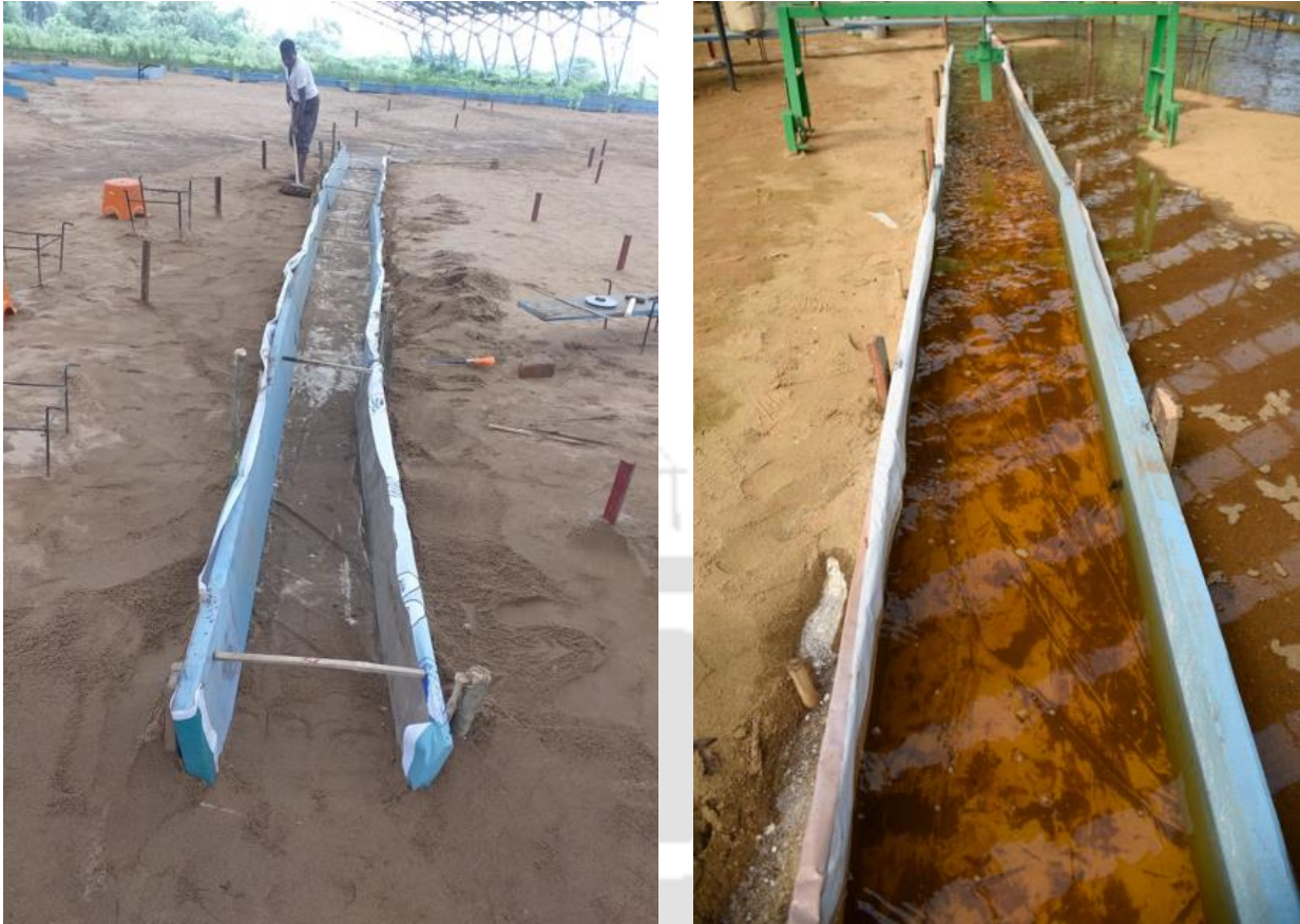
Figure 7.2 Construction of Dredging Channel in Physical Model
