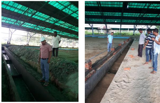
Construction of Arrangement for Exit of Water
