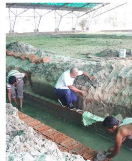
Construction of Arrangement for Exit of Water
