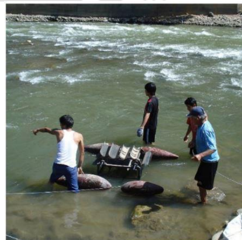
Figure 6-3 Installation of Schottel hydrokinetic river turbine
