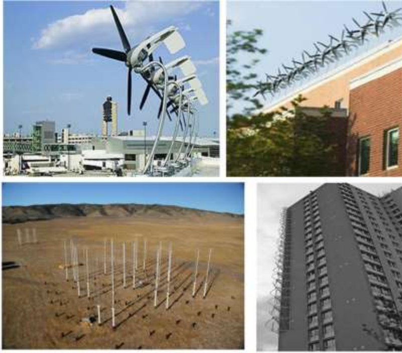
Fig. 2.7. Cluster arrangement of small wind turbine (Reproduced with permission from Casini et al. 2016; Liu et al. 2019; Dilimulati et al. 2018)
