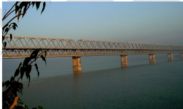
Fig. 2.1. A photographic view of the Saraighat Bridge
