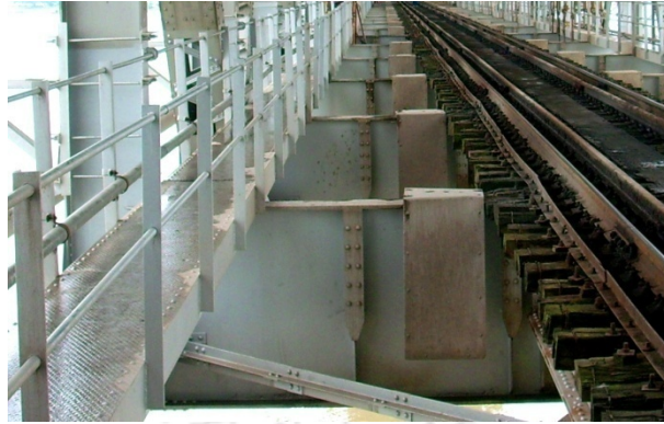
Fig. 4.16. View of rail-level cross-girders
