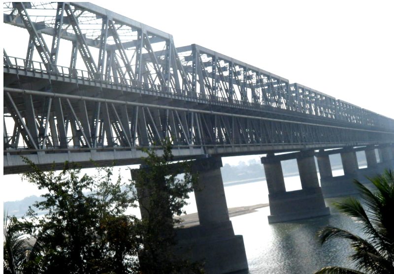
Fig. 3.1. A photographic view of the Saraighat Bridge
