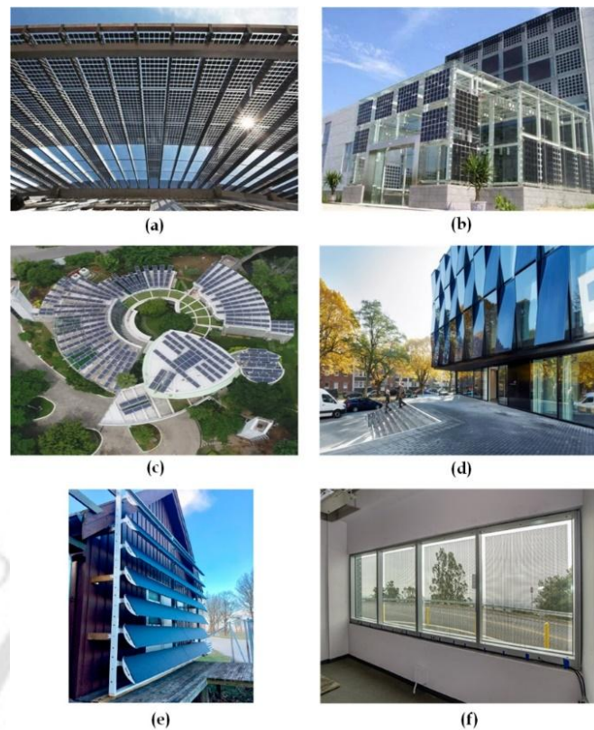
Fig. 1.4 Different form of BIPV application in buildings. (a) BIPV skylight system [15] (b) BIPV solar facades system [15] (c) BIPV rooftop system at Indian Green Business Centre (IGBC) - Hyderabad, India (d) Solar PV facades in NEW-Bauhaus Building, Germany [16] (e) PV as blinds integrated to building [17] (f) PV based windows at FLEXLAB, Solaria BIPV [18]
