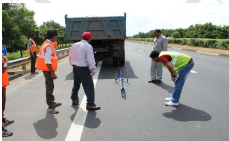
Photo 4.1 Benkelman beam deflection test at NE-1GJ01 at Km. 14.50
