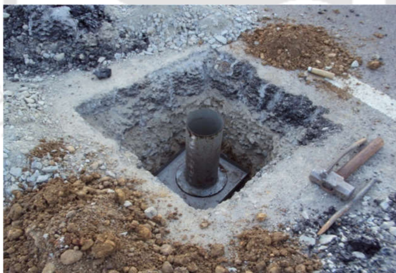
Photo 4.6 Observation of test pits
