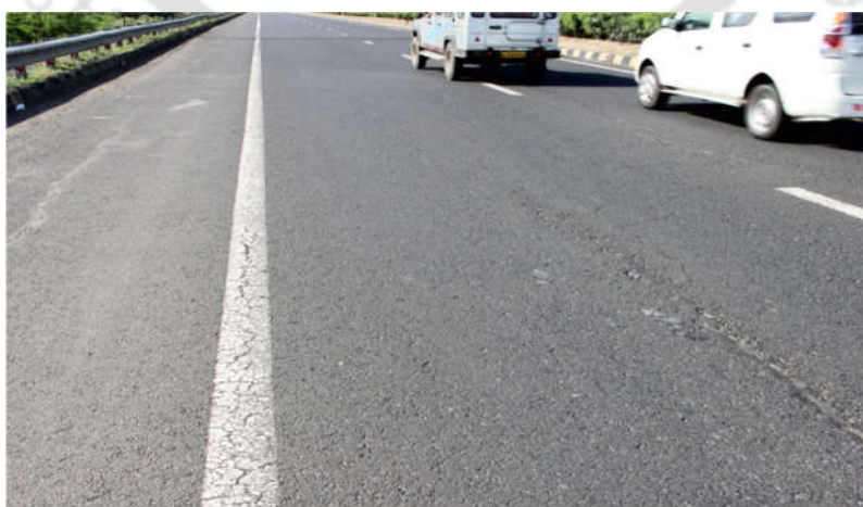
Photo 4.2 Surface condition evaluation on pavement section NE-1GJ at Km. 32.00
