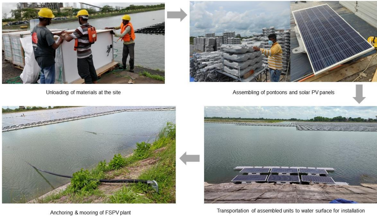
Figure 3.2. Installation activities on land (Image source: author)
