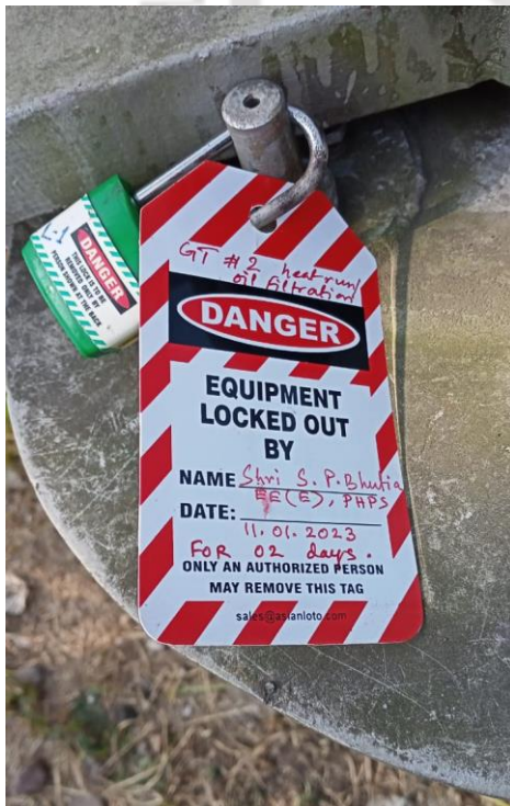
Figure 6.7. Photographs showing Lock Out Tag Out (LOTO) for electrical safety (image: author)
