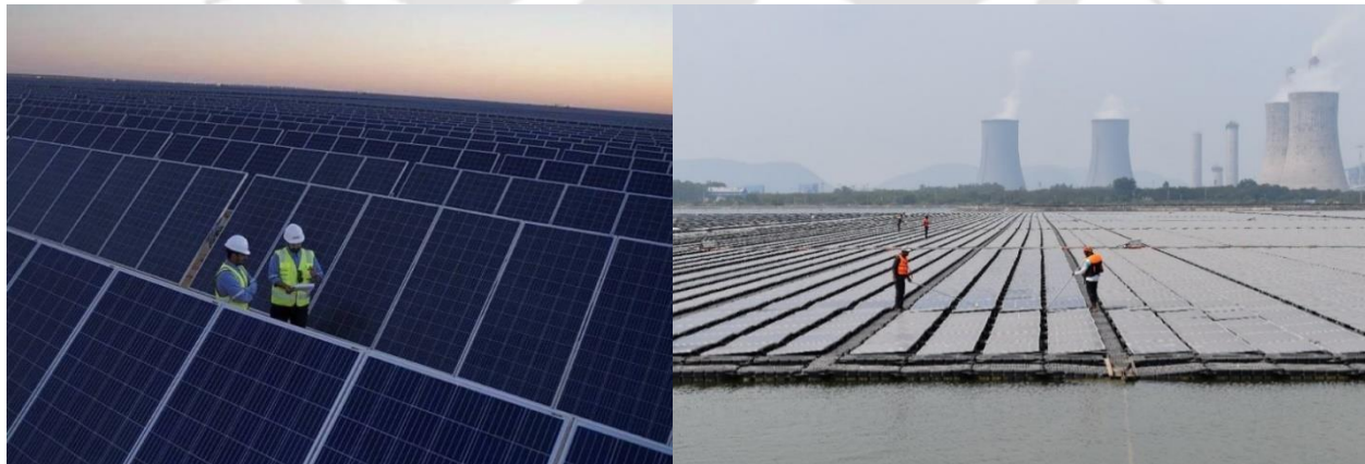
Figure 5.2. Workers (left) engaged in maintenance at the 300 MW solar farm at Saudi Arabia and FSPV workers (right) engaged in cleaning of solar panels at the 25 MW floating solar project in India. (Image source: authors)
