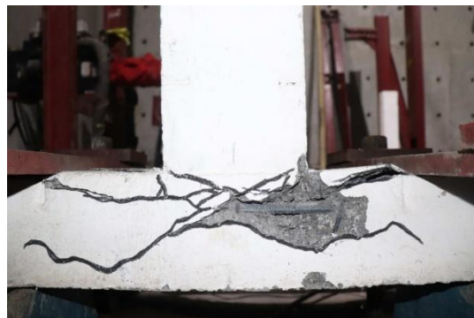
Figure 6.11 Evolution of damage in Seismic specimen (S)
