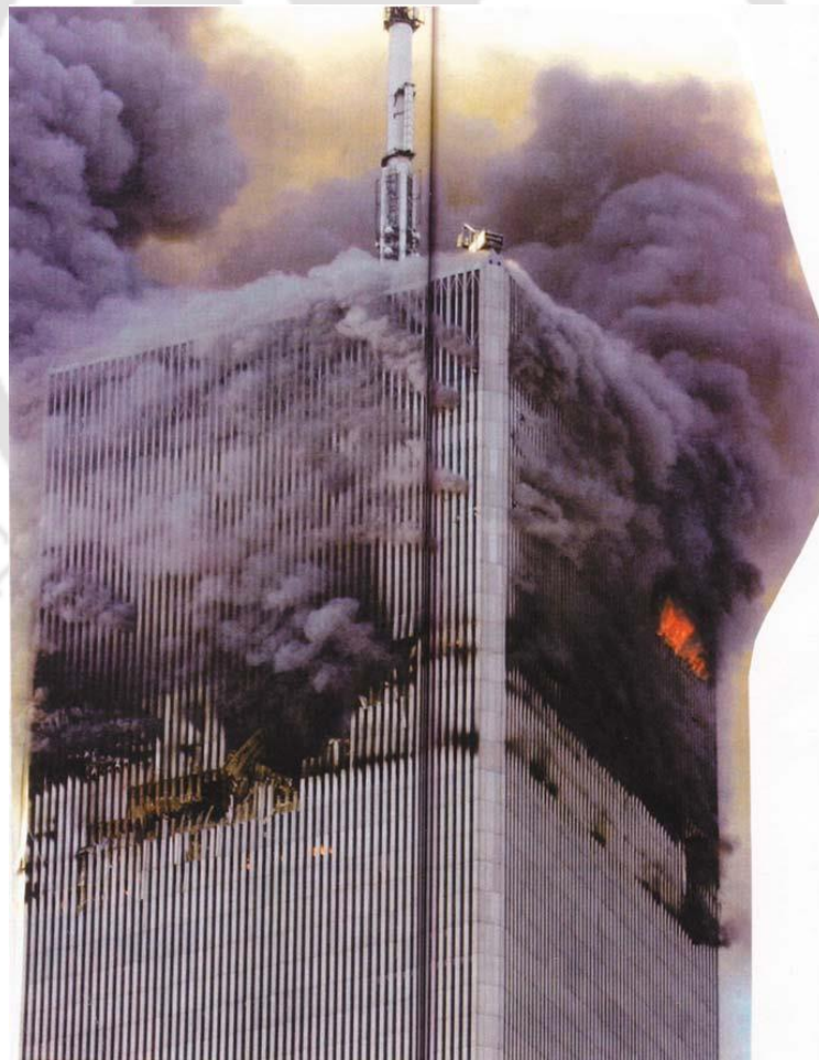
Figure 2.2 World Trade Center (WTC) Tower with antenna-Blast and collapsed scenario: Tower I (Bangash 2006)
