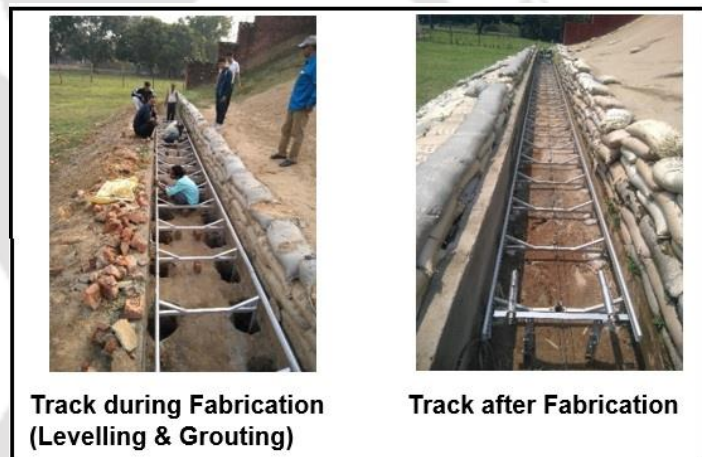
Figure 3.2 : Photos depicting Track, during & after Fabrication
