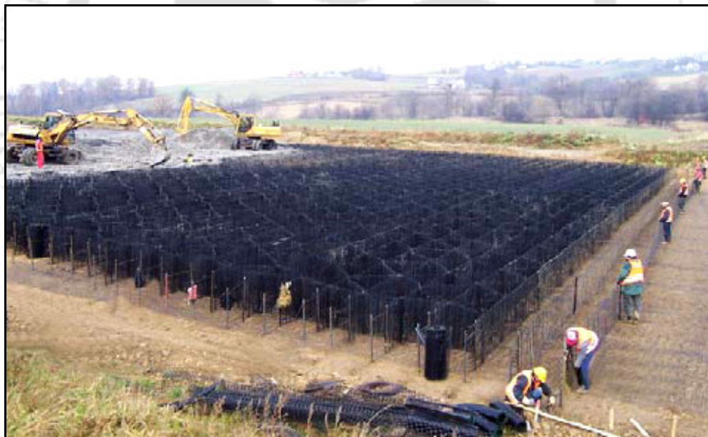
Photo 1.4 Construction of geocell mattress nearing completion (Kawalec et al., 2006)
