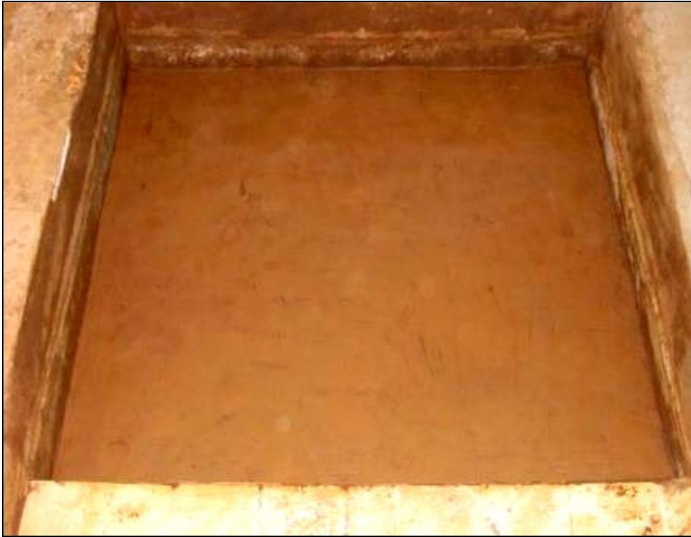
Photo 3.4 View of the prepared clay subgrade
