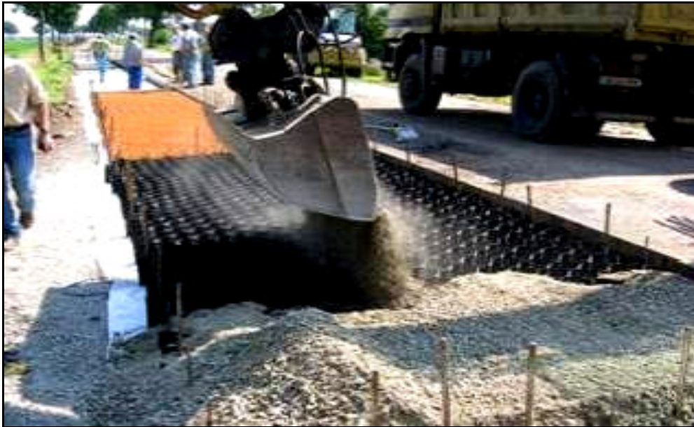
Photo 1.2 Installation of geocell in the field (Emersleben and Meyer, 2008)
