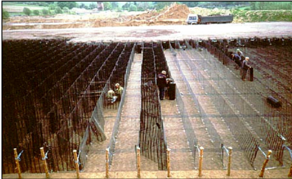
Photo 1.3 Construction of geocell mattress in progress
