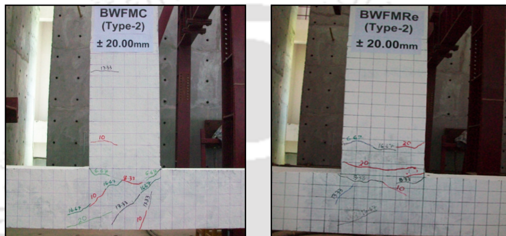
Fig. 3.9 Initial appearance of cracks for BWFM specimens under loading type-2
