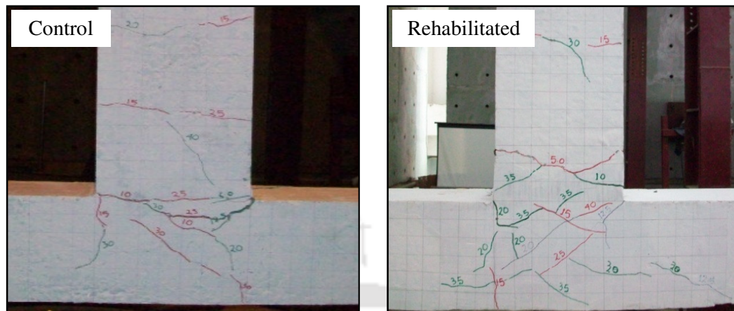
Fig. 4.4 Appearance of cracks for BWSL specimens under loading type-2 corresponding to peak load
