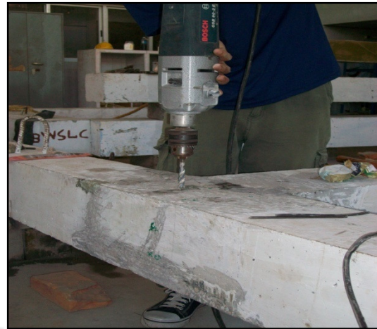
(b) Drilling holes along cracks
