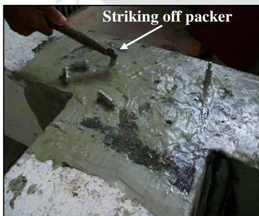
(e) Removing of installed packers
