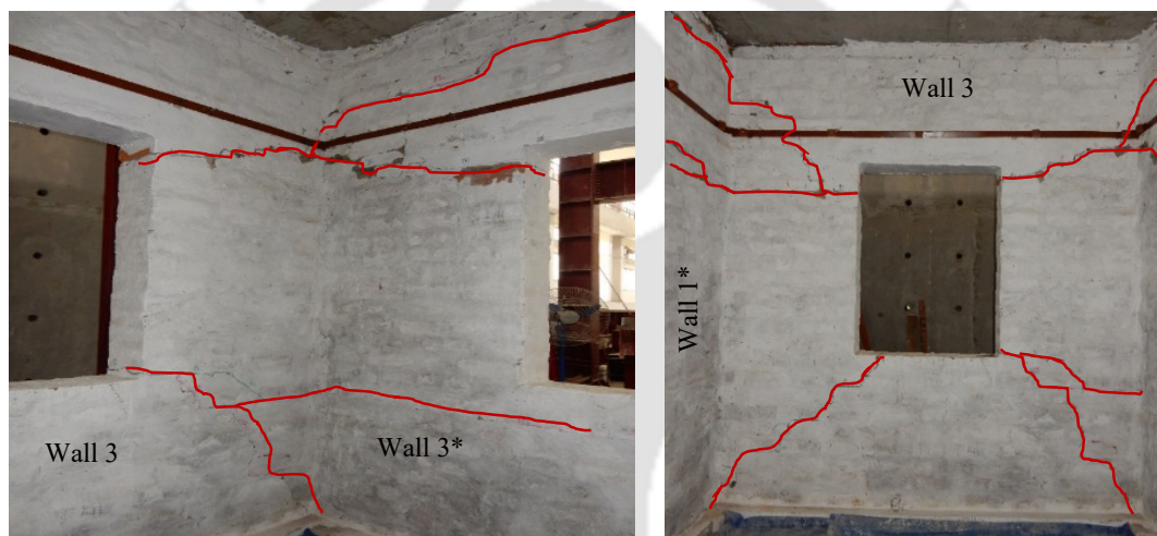
Figure 5.12. Damage observed in different walls inside Model 1 during the lateral load testing.
