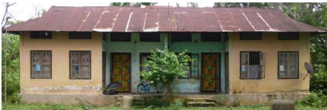
Figure 1.5. An unreinforced brick masonry house with GI sheet on roof.
