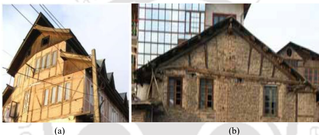
Figure 1.8. Traditional masonry for proven earthquake resistance: (a) Dhajji-dewari system of timber-laced masonry for confining masonry in small panels, (b) Taq system of embedding timber logs in thick walls (Rai and Murty, 2005).
