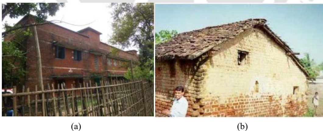
Figure 1.3. Type of URM buildings: (a) Unreinforced brick masonry with reinforced concrete slab, and (b) Unreinforced brick masonry with pitched clay tile roof (Kumar, 2002).
