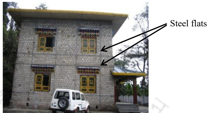
Figure 1.9. Excellent performance shown by retrofitted Archive building during 2006 Sikkim earthquake (arrows indicate locations of steel flats used to retrofit the building after 1988 Bihar-Nepal earthquake) (Kaushik et al., 2006).
