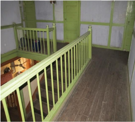
Wooden flooring, first floor
