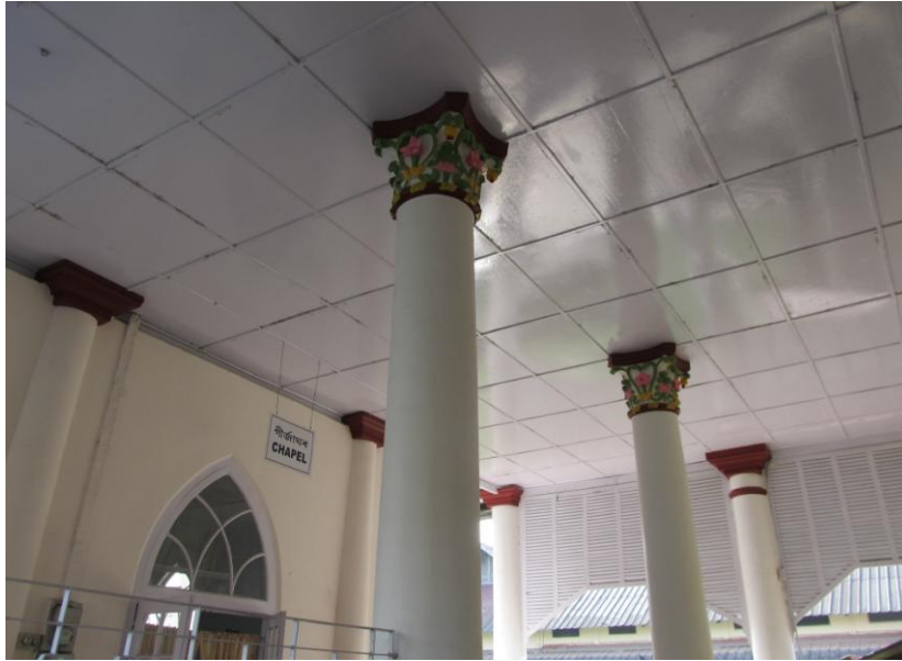
Decorated capital on columns, Church, Satribari Christian Hospital
