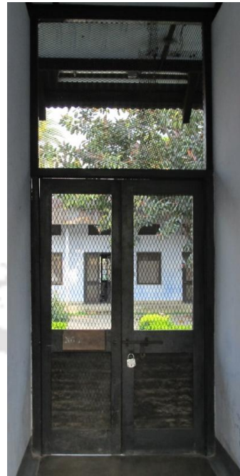
Entrance door to the Hostel of the Nursing College
