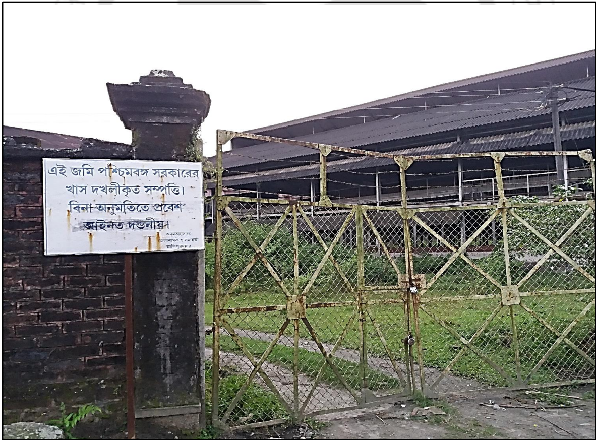
Photograph 8: Abandoned Factory of Patabari Tea Estate, Alipurduar
