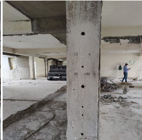
(b) A column after drilling bore holes
