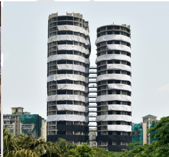
(d) Residential towers after charging with explosives, just before demolition
