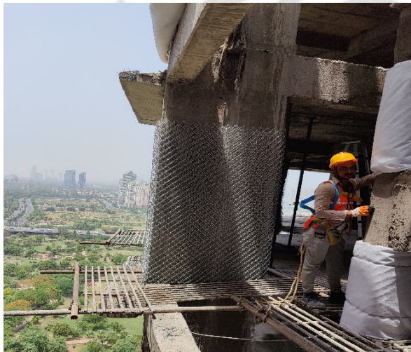
(c) Wrapping of columns with chain link fence and geo-textile fabric
