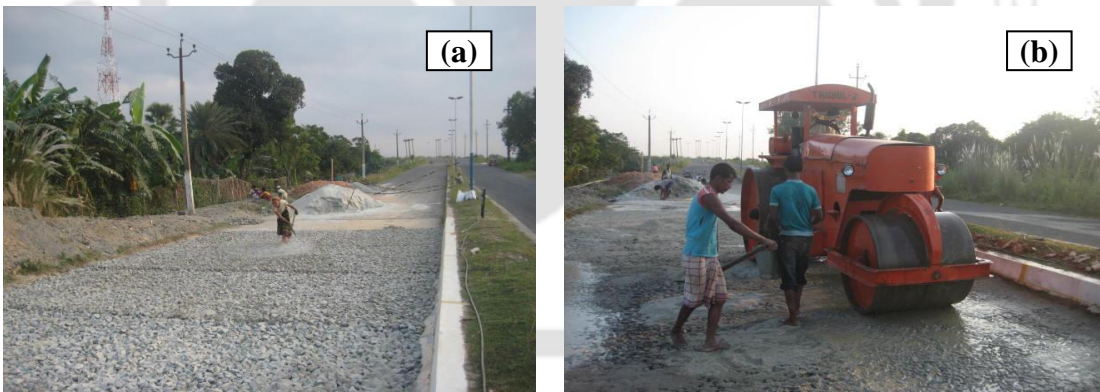
Figure 3.8: a) Laying and b) Compaction of the WBM course.
