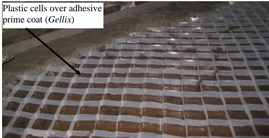
Figure 3.13: Casting of the PCCBP overlay over adhesive prime coat ( Gellix ).
