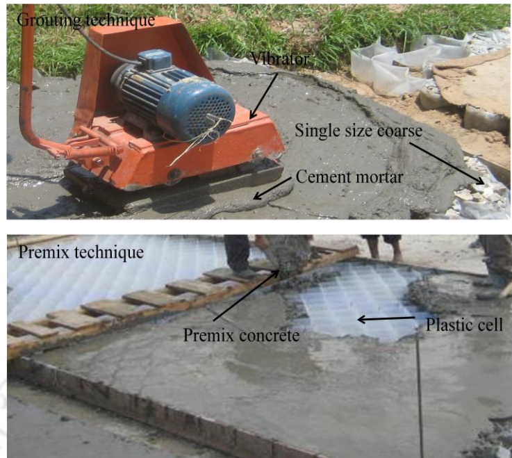
Figure 3.3: Comparison between grouting and premix technique for construction of PCCBP pavement.
