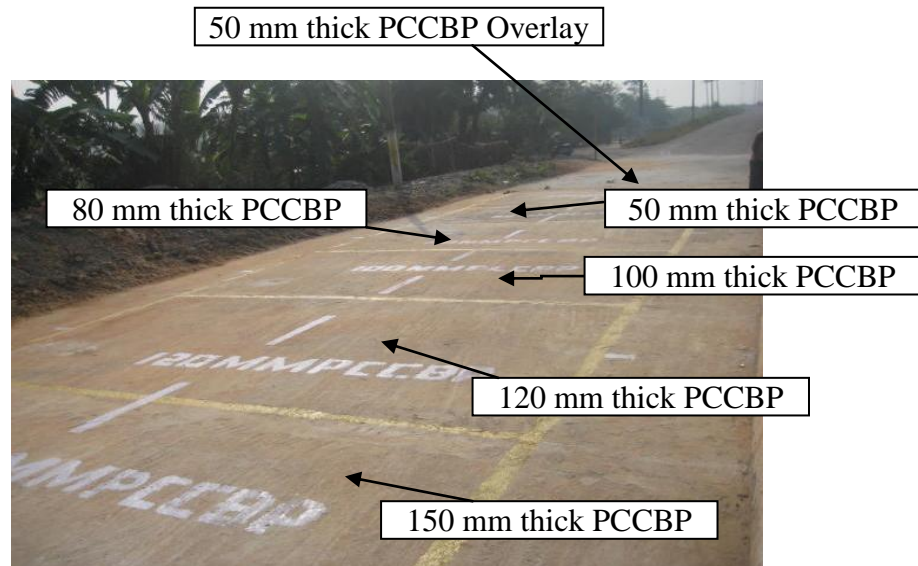
Figure 3.15: Completed PCCBP test road with markings for different test sections.
