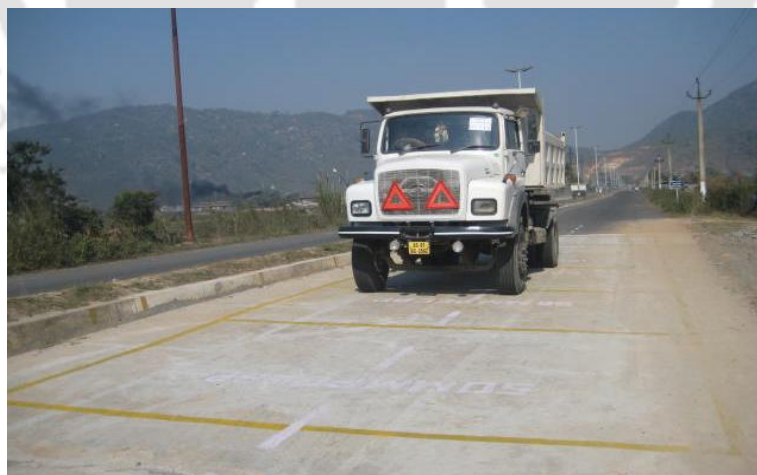
Figure 3.18: Completed PCCBP test sections opened to regular traffic.
