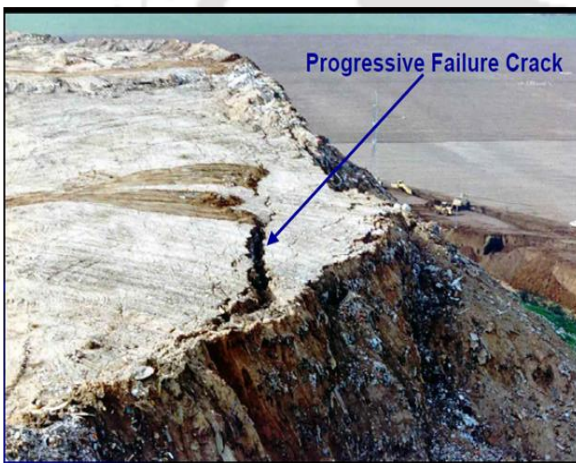
c. 1997 Hiriya landfill slope failure (Isenberg 2003)
