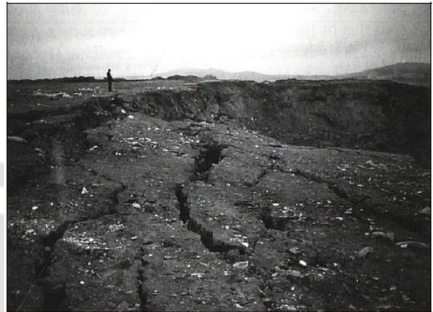
b. Tension cracks on top of landfill and steep backscarp in MSW after slope failure (Kocasoy and Curi 1995)
