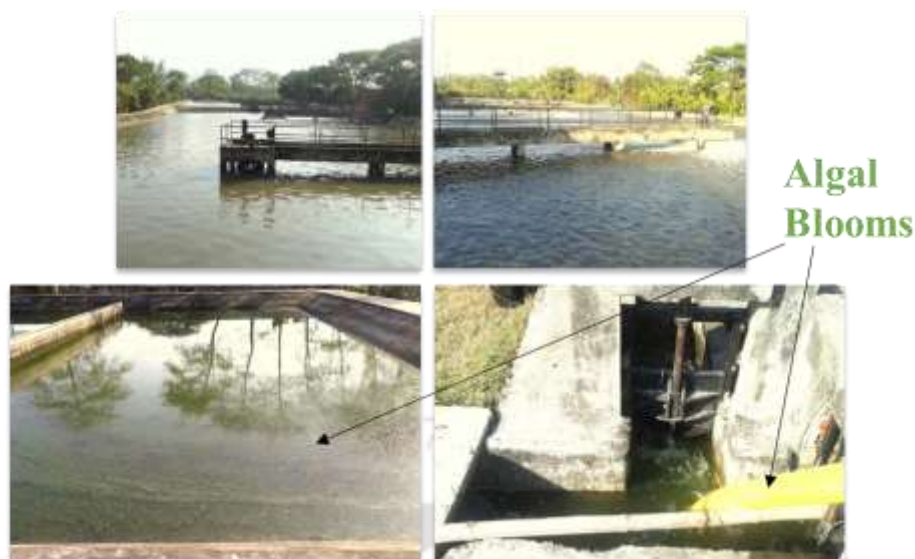
Fig. 3.1. Sewage treatment plant, located at the Indian Institute of Technology Guwahati, India.
