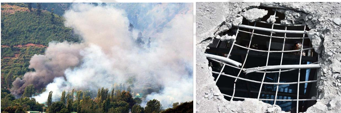
Figure 1.2 Artillery shelling in Uri (left) (Hassan 2018) and damage due to shelling (right)
