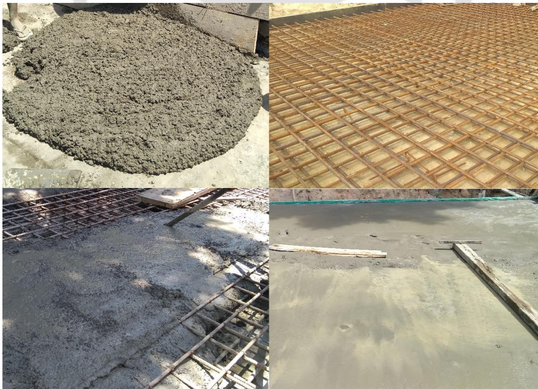
Figure 10.13 Photographs of high strength concrete slab during casting.
