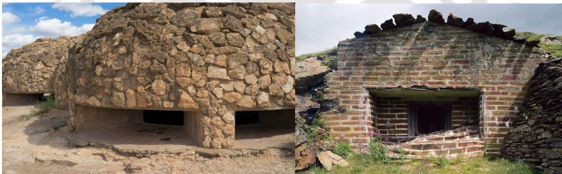
Figure 1.9 Stone (left) and Brick (right) Bunkers (Fabrizio 2004; Speier 2013)
