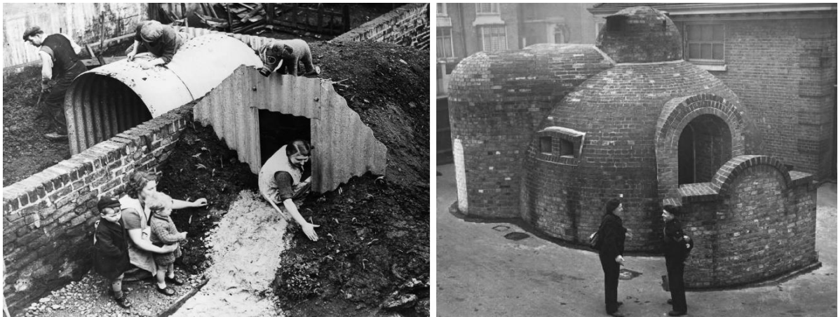
Figure 1.12 Anderson shelter (Reddit 2015) (left) and Igloo-shaped Brick shelter (Harlow 2018) (right)
