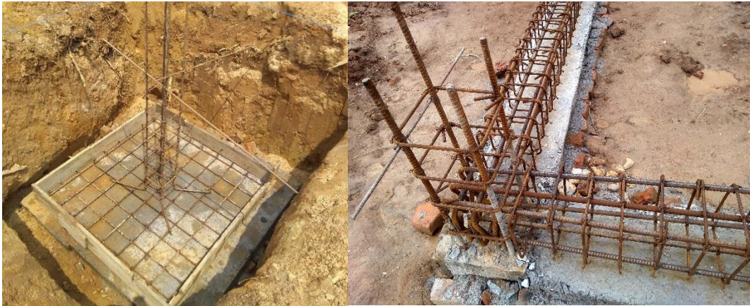
Figure 10.11 Photographs of laying of footing (left) and tie beam (right)
