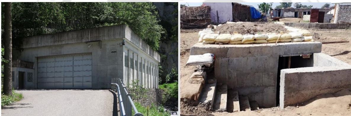
Figure 1.13 Swiss government bunker near Kandersteg in canton of Bern (Kecko 2015) (left) and Civilian bunker in Rajouri village, India (The Statesman 2020) (right)
