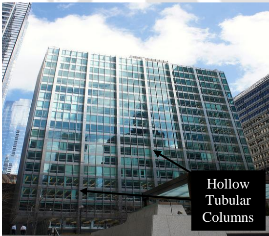
(c) Inland Steel Building in Chicago (Courtesy: Galinsky)
