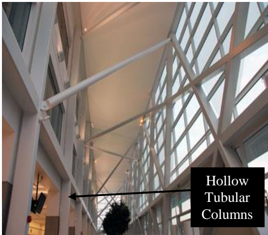
(a) Transit terminal in Wisconsin (Courtesy: SSEF)
