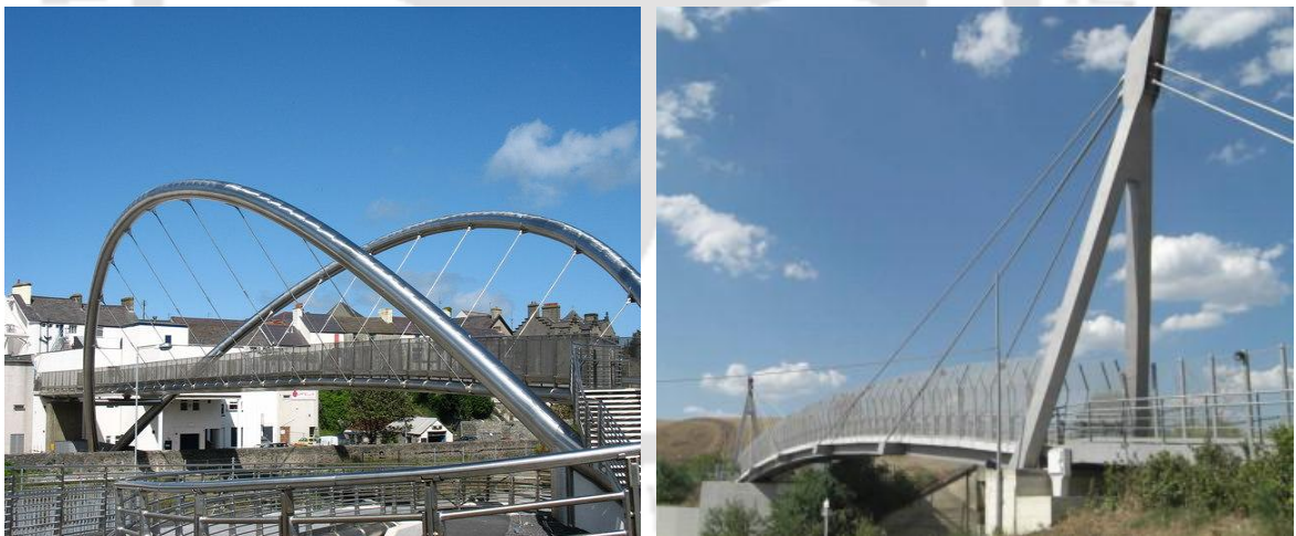
(a) Celtic Gateway footbridge in UK (Courtesy: Wikimedia)
