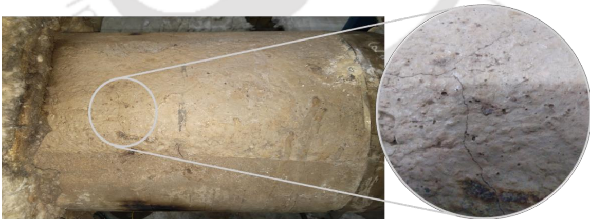
Figure 4-20. Photographs of minor crack formation in the CTES module.
