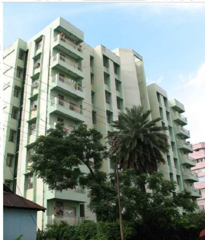
Fig. 4.2: Photograph of nine-storey building (photo courtesy Borsakia et al. (2010))
