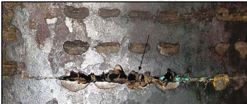
Fig. 1-9. Washout was observed on the drill pipe body
