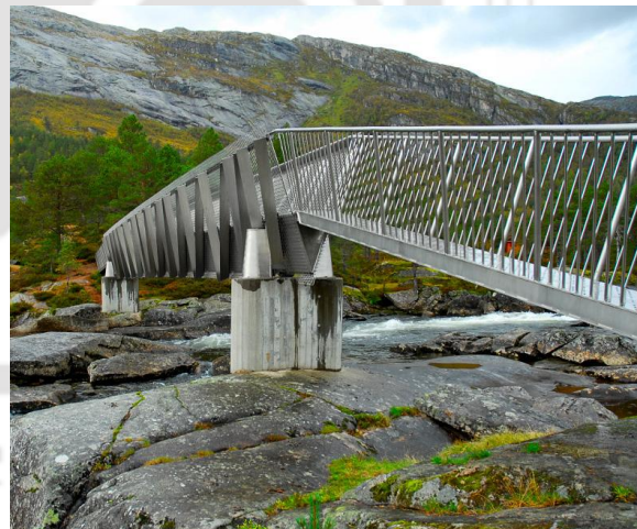
Figure 1.7: Likholefossen Bridge in Norway ( amazonaws.com )
