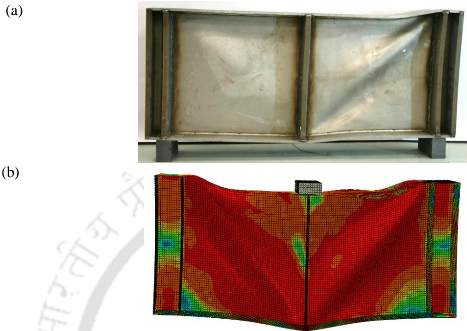
Figure 4.3: Typical failure mode of 3PB specimen of LDSS plate girder (I-600×200×12×8) showing (a) Experiment (Saliba and Gardner, 2013b) (b) FE
