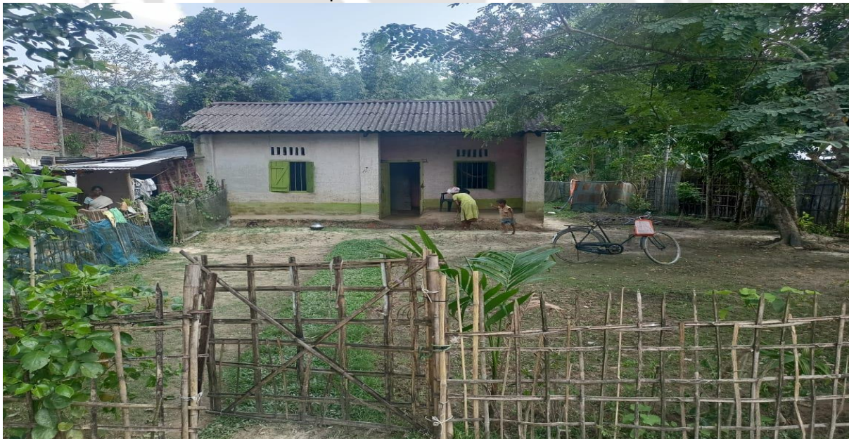
Picture 4.3: A view of the workers' quarter
