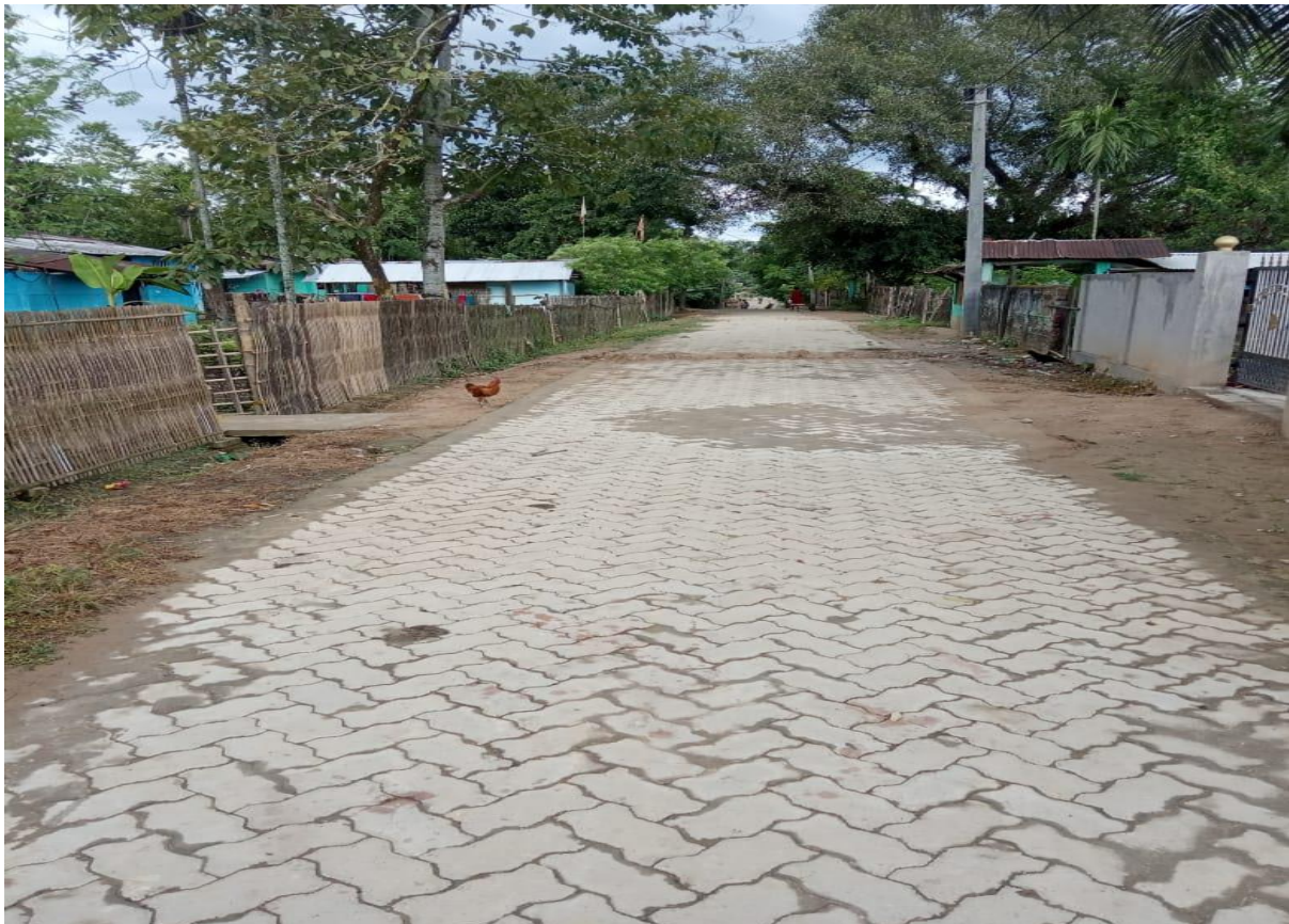
Picture 6.1: A newly constructed road in the Coolie line
