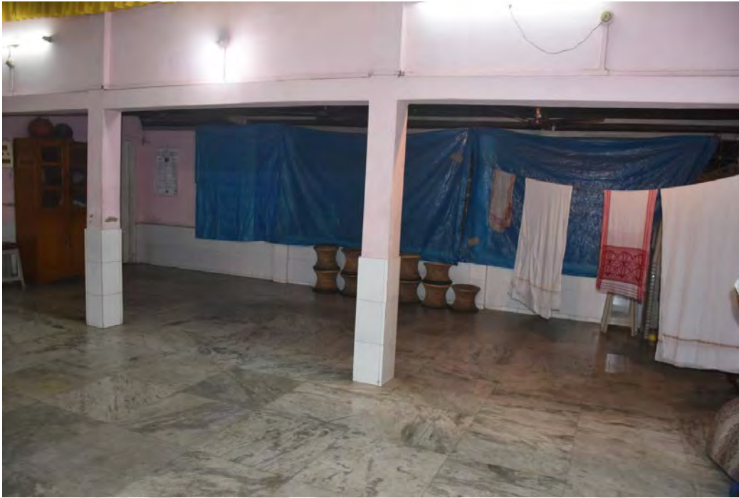
Fig. 5.3: Square plain pillar at Akasipath Naamghar
