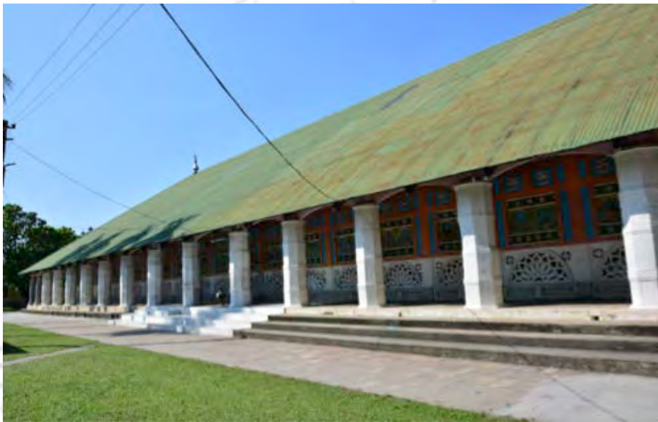
Fig. 4.3 (a): Exterior of Naamghar (South side) in Barpeta Satra (Photograph: Researcher)
