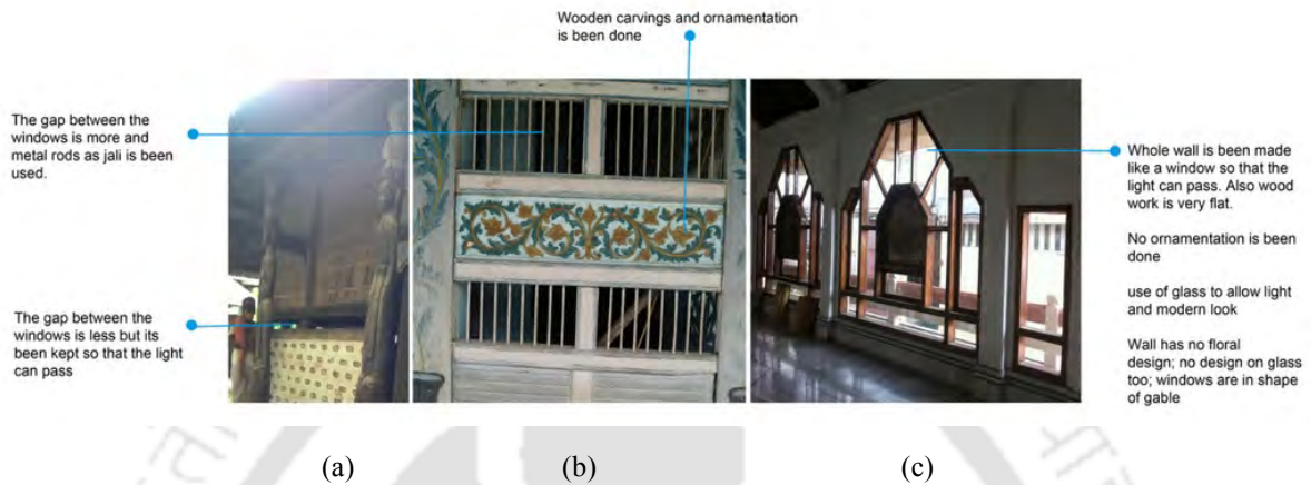
Fig 4.79: Comparison of windows of Naamghar in (a) Sarbogh Naamghar Garakhia Gosain Than , 100 years (Rural) (b) Ramdiyar Naamghar , 75 years (Semi-urban) and (c) Zoo Road Naamghar , 18 years (Urban area) (Illustration: Researcher)
