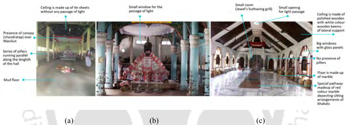
Fig 4.81: Comparison of Prayer hall of Naamghar in (a) Sarbogh Naamghar Garakhai Ghai Gosain Than , 100 years (Rural) (b) Ramdiyar Naamghar , 75 years (Semi-urban) and (c) Zoo Road Naamghar , 18 years (Urban area) (Illustration: Researcher)
