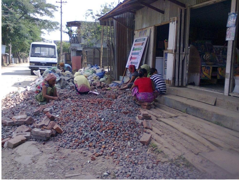
Figure 7: Women engaging in construction work
