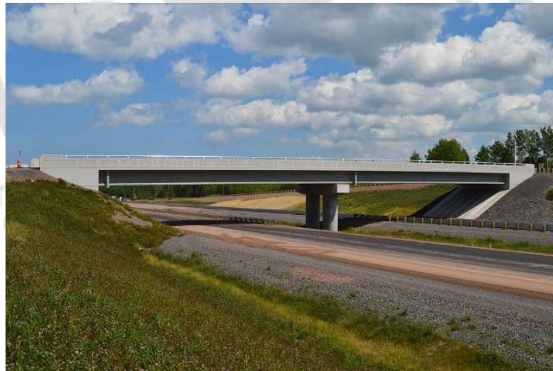
Fig. 1.1 Integral Abutment Bridge (Addington Forks Underpass, Canada)
